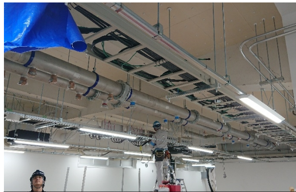
Piping and cabling hang from the ceiling
